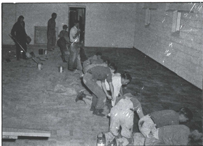
FINISHING AUDITORIUM- GYMNASIUM FLOOR, DEDICATION WEEK
