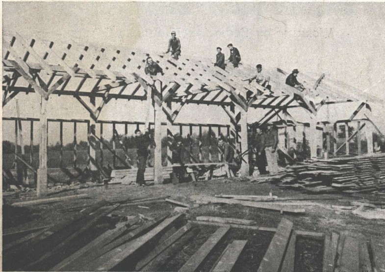
STUDENTS CONSTRUCT AN IMPLEMENT HOUSE
