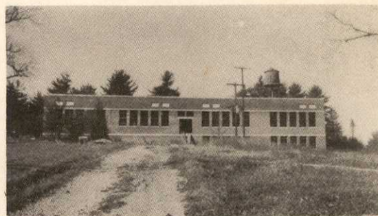
New Elementary Building
